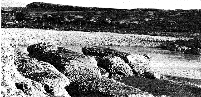
23. REMAINS OF BARRAGE BELOW PIERS OF ARRAJĀN BRIDGE, ON RIGHT BANK
